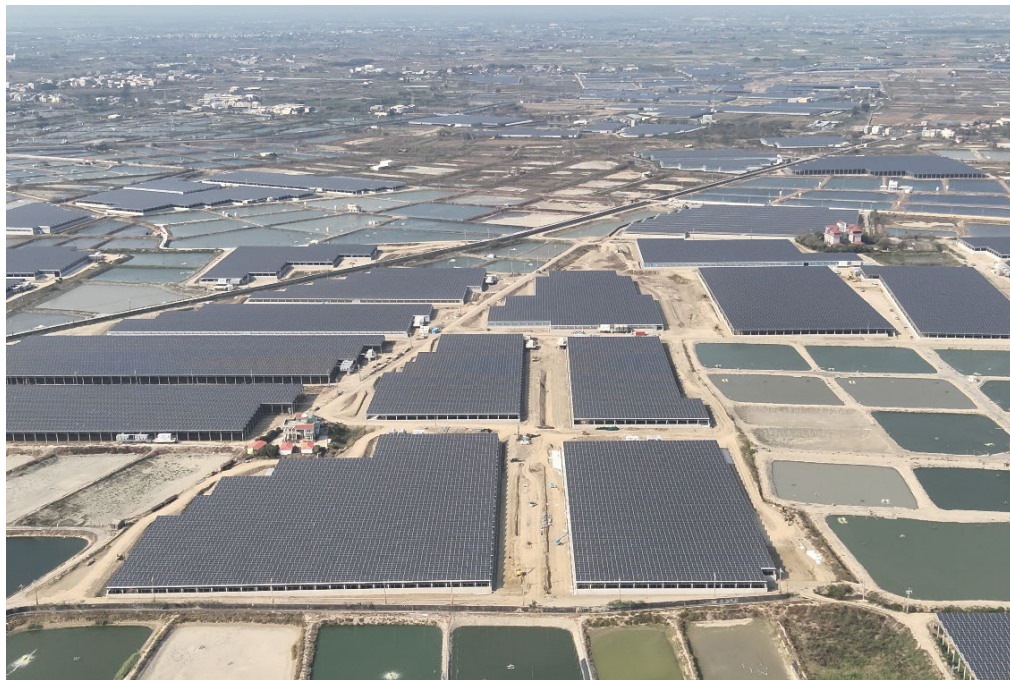
<Aerial Photo of the Phase 1 site>
